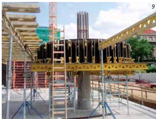
Fig. 10 Completed formwork of the ceiling with heads above the columns
