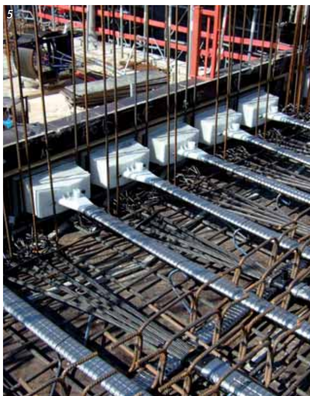
Fig. 5 Stressing and dead-end anchorages of the SO 6-4 system
