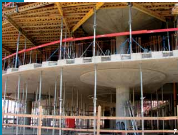
Fig. 8 Tendon placing of the 3rd floor
