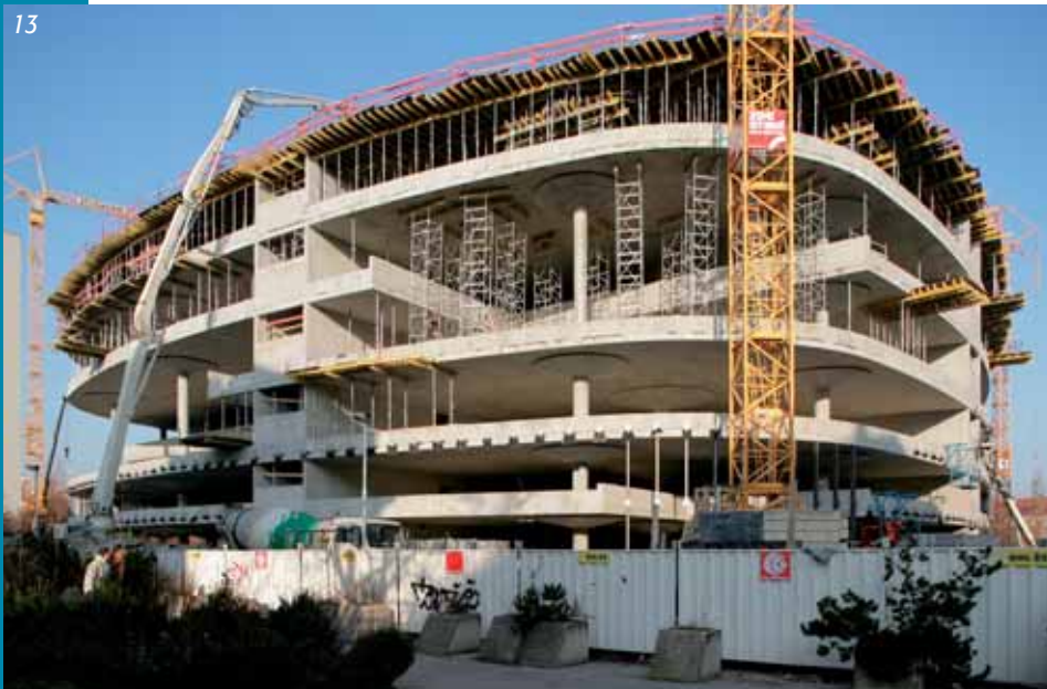
Fig. 13 Library building during concreting of the top ceiling
