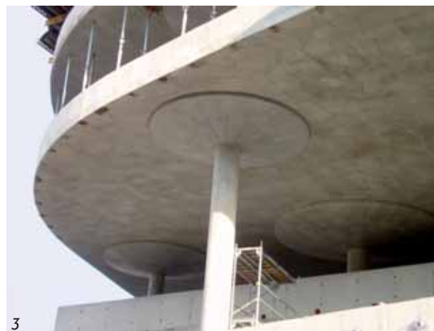
Fig. 3 Columns with heads in the peripheral part of the ceiling
