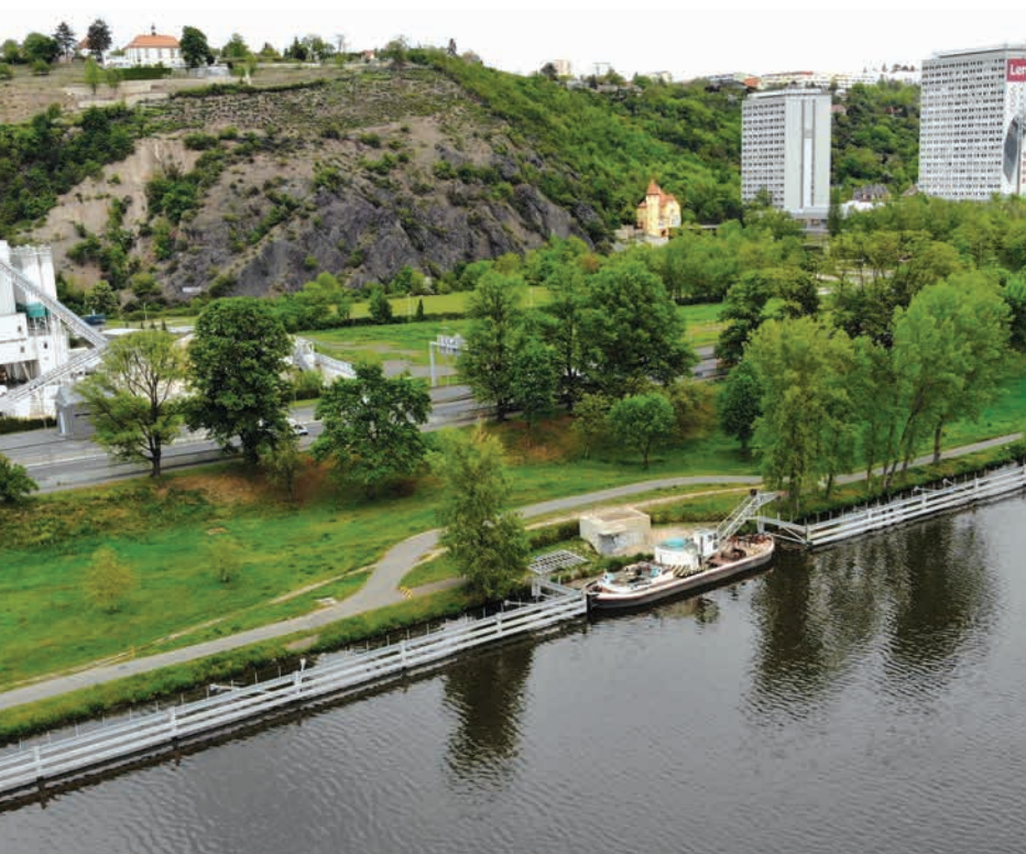
Betonárna Libeň Concrete Mixing Plant Libeň
